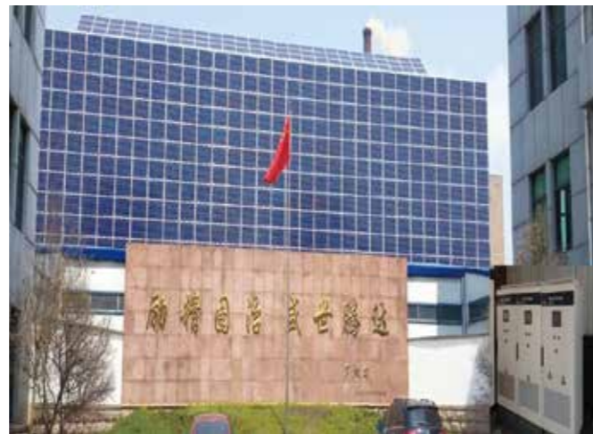
ANBF-1000K for 5.5MW solar power station at Longkou Shengda Glass Products Co., Ltd
