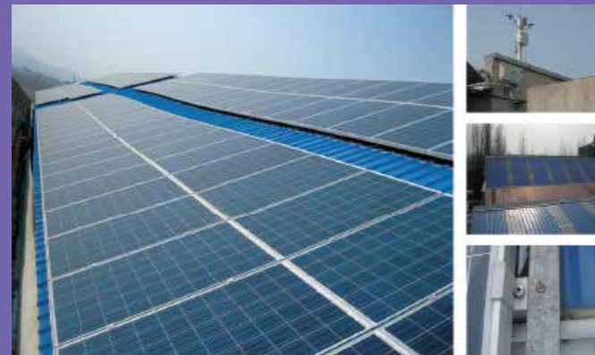
92kw Distributed PV Projects at Jinan This project is set up at factory rooftop of Jinan Runtong Steel Wire Brush Ltd. The rooftop is color steel tile and face south. Total area is about 660 sqm. Power generation is for own use and the rest power is fed into the grid.
