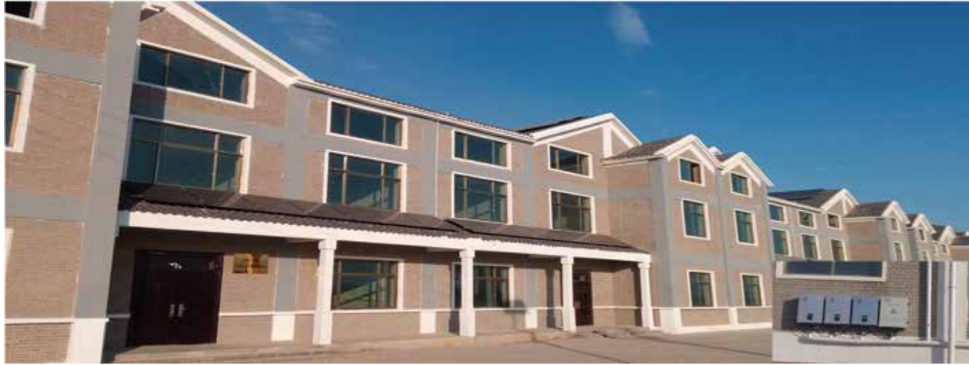
HF series for first 226.8KW grid-connected solar power station of Hanergy at Yumen
