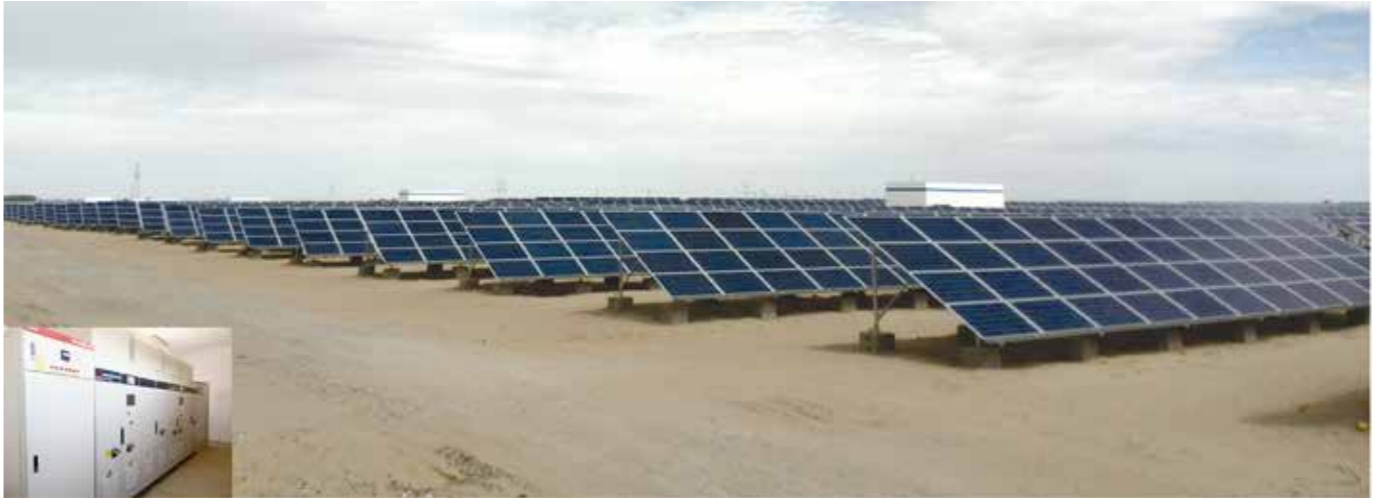
ASP-500KTL for 65MW solar power station at Huaneng Golmud
